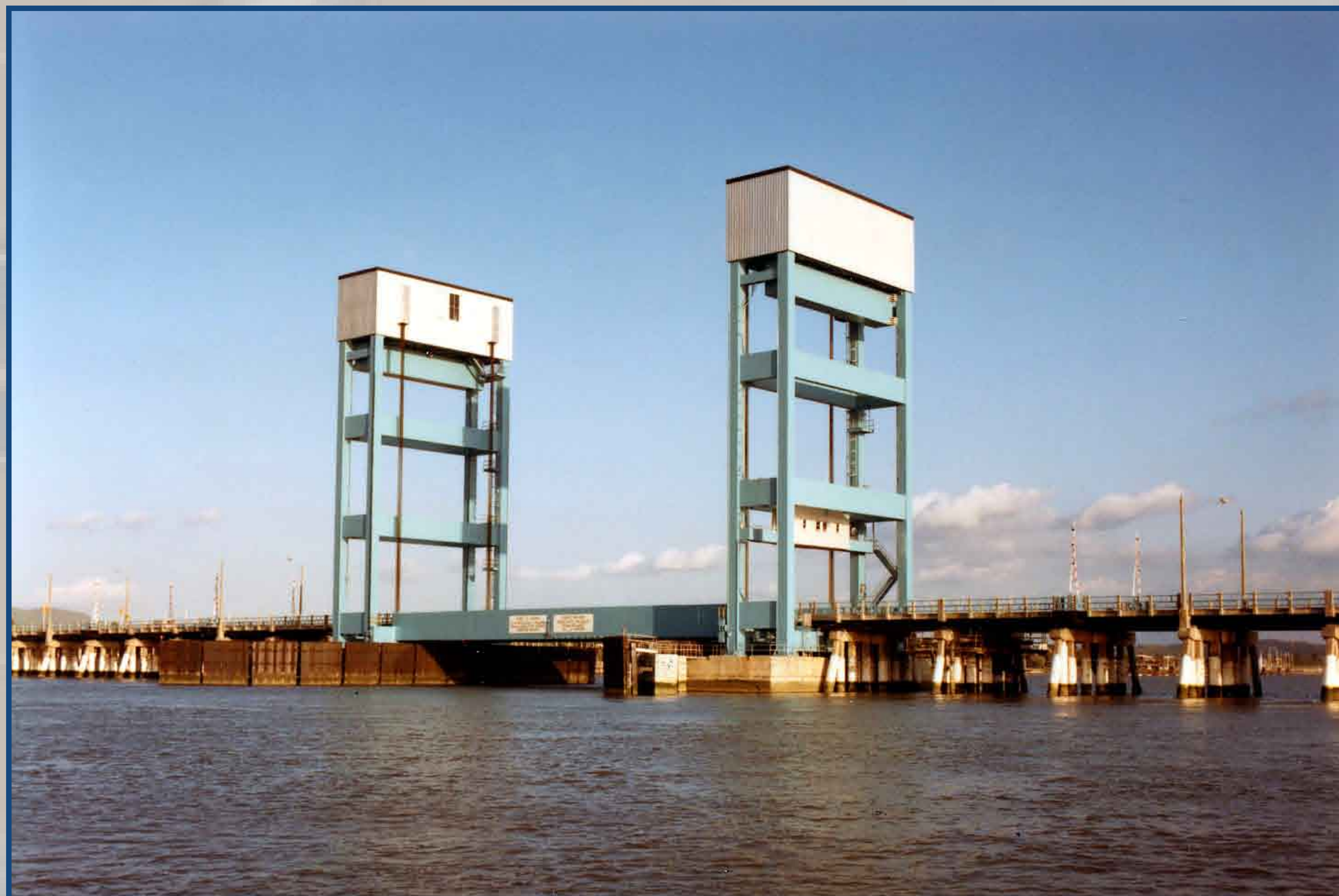
Mare Island Bridge, Valejo, CA
