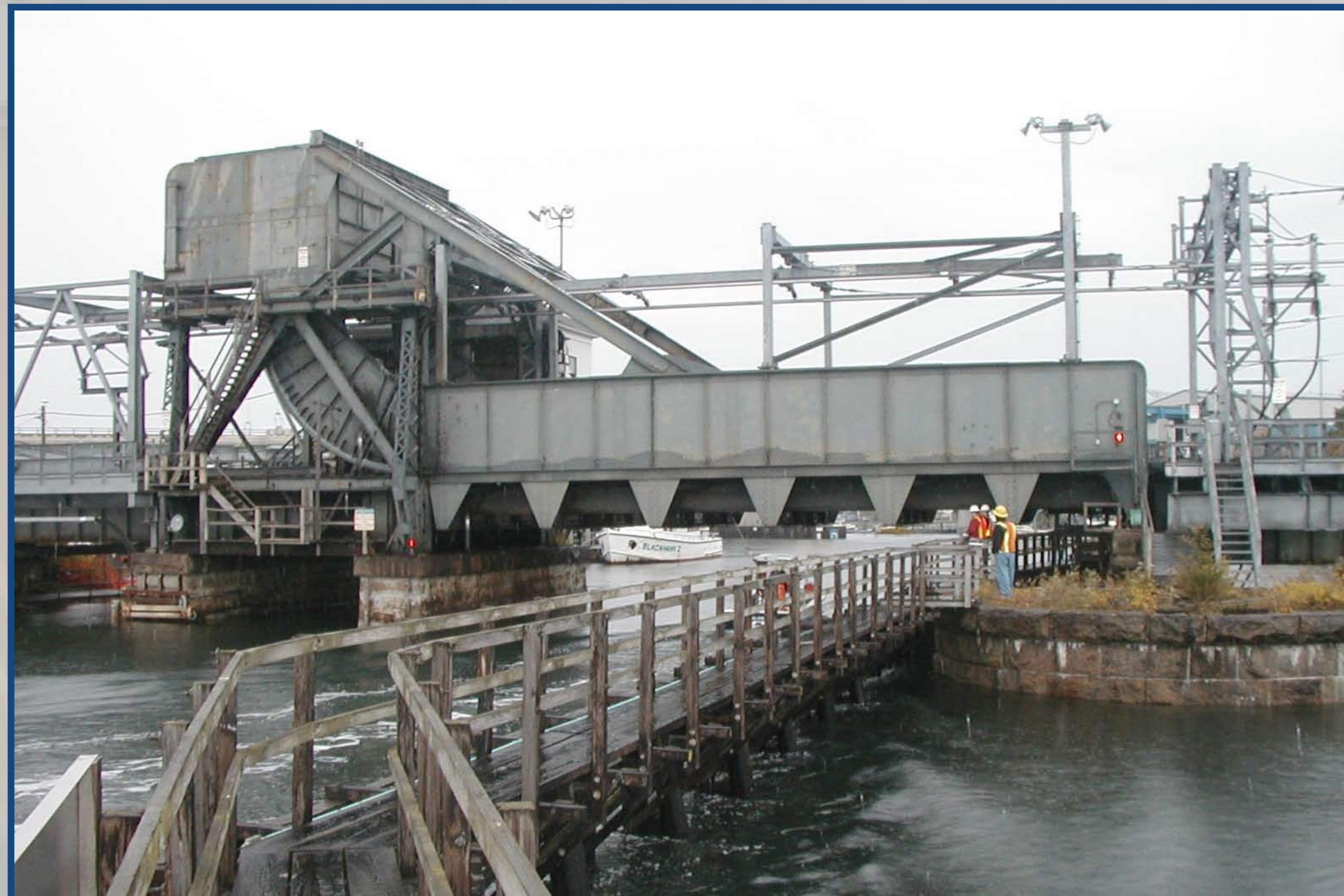
Niantic River Railroad Bridge for Amtrak, Waterford, CT
