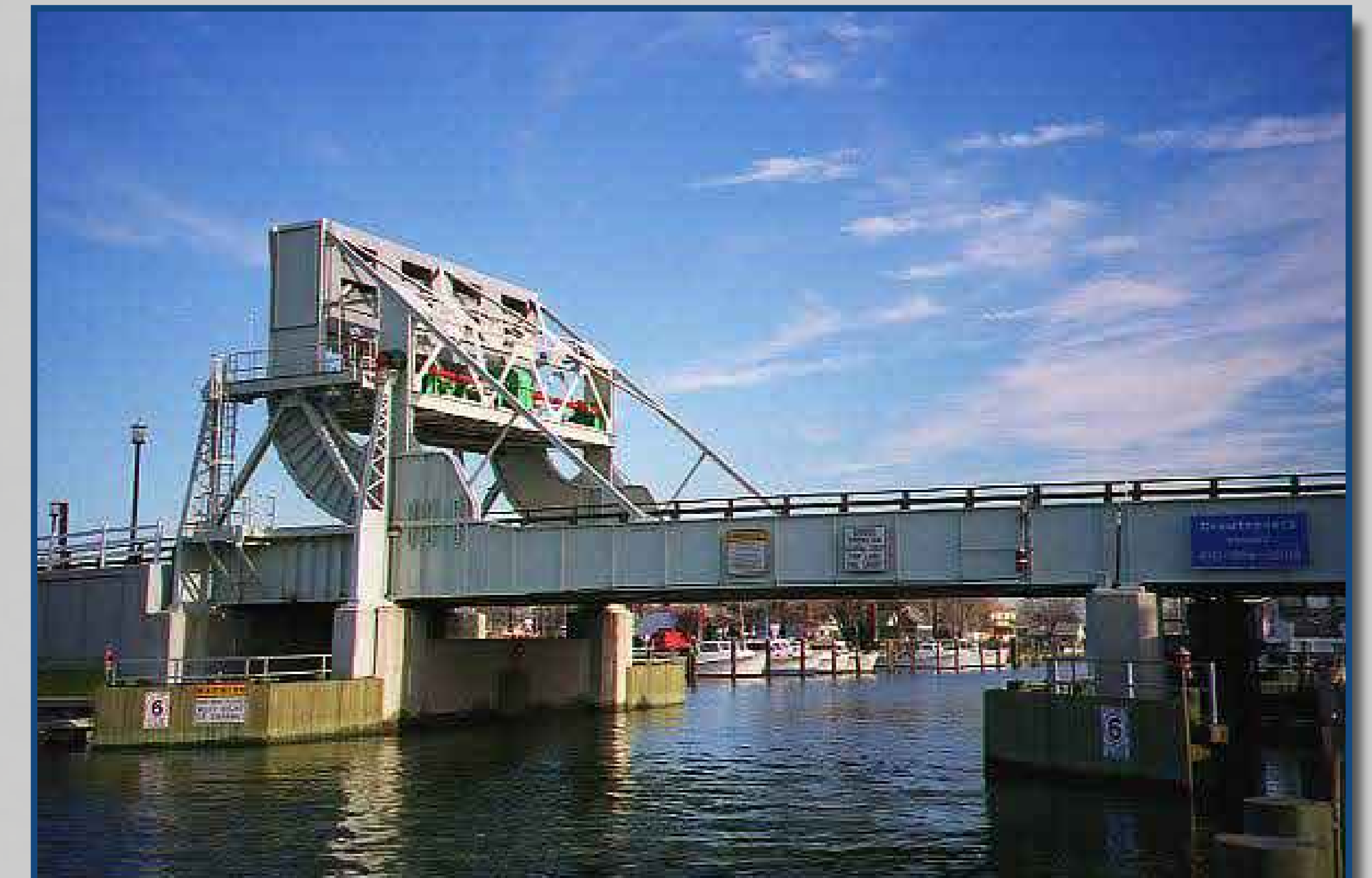
Tilghman Island Bridge, Tilghman, MD
